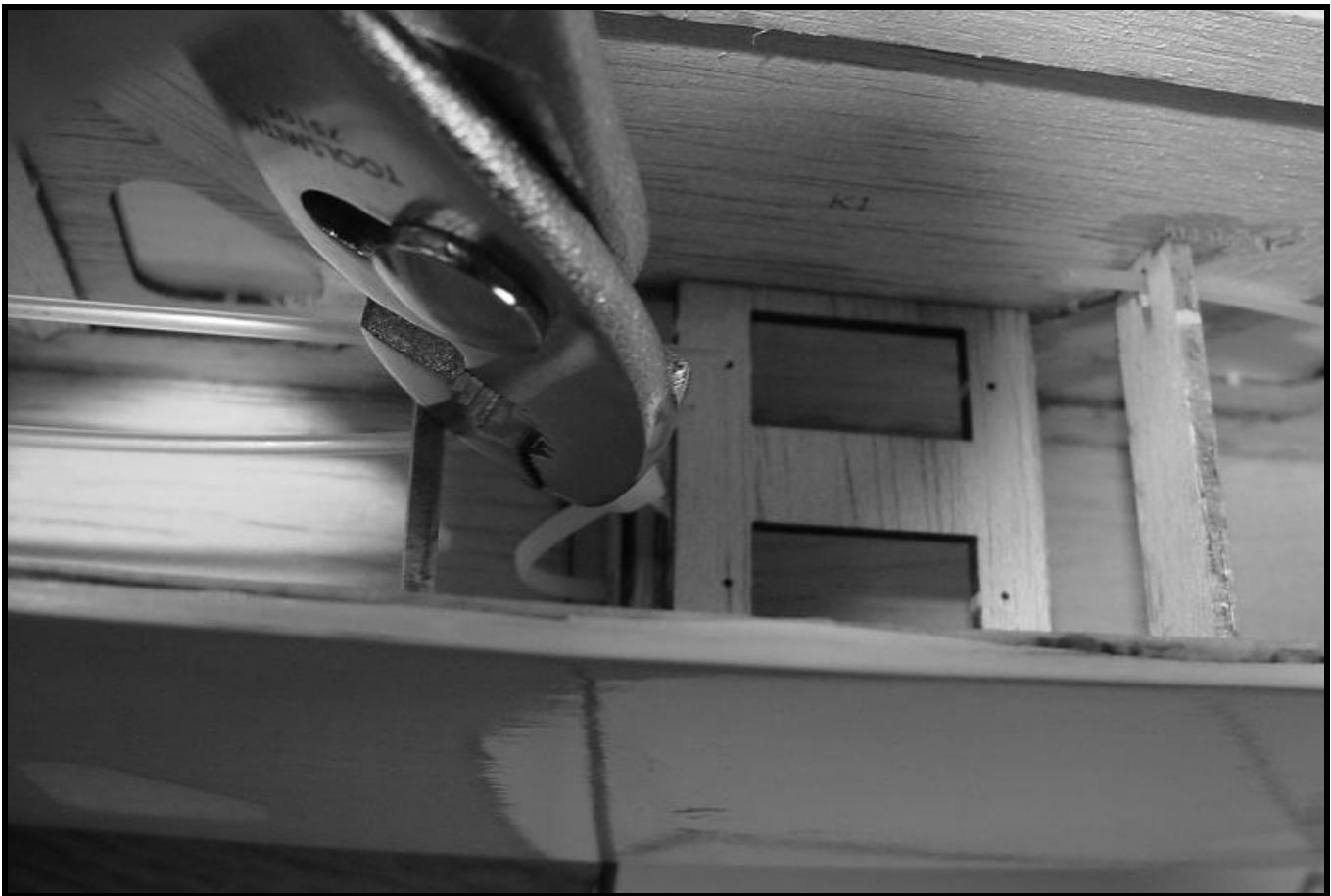
Photo illustrating installation of Zip-tie fastening to fuselage's main landing gear pocket
